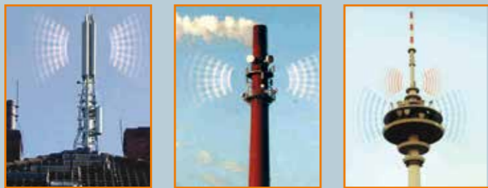
Mobile phone senders on roofs, chimneys and television masts
